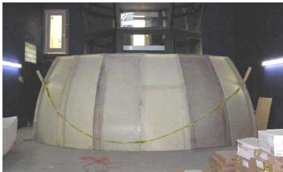
Figure 5 Assembly of the Upper Part of the Dome Screen
