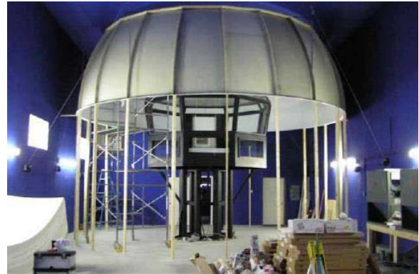
Figure 6 Upper Dome Section During Installation
