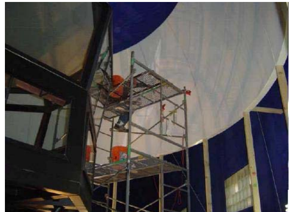
Figure 7 Caulking and Painting the Dome Screen.
